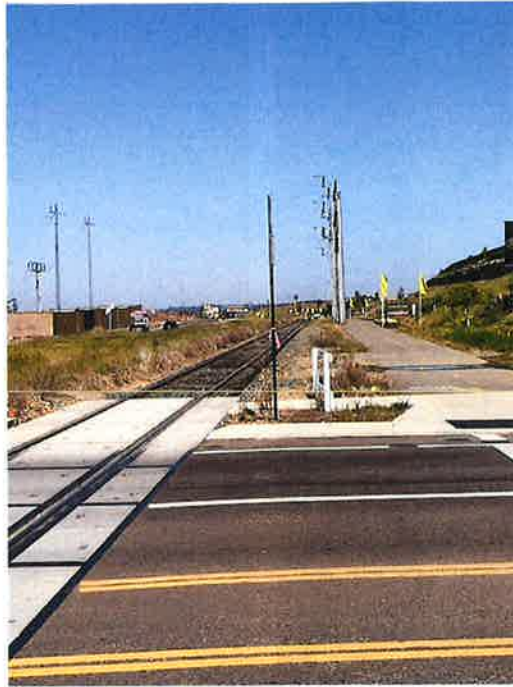
Sign post installed within 8' 6" of track center creates a contact hazard.
